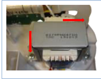
Unscrew the transformer
